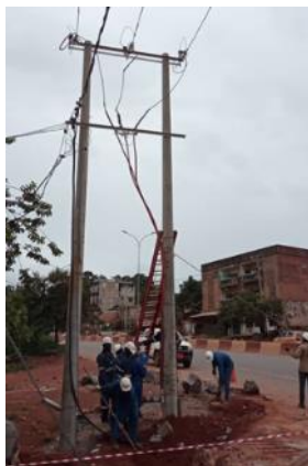
Yaoundé: Replacement of critical wooden poles with concrete poles in Emana and its surroundings
