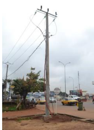
Yaoundé: Replacement of critical wooden poles with concrete poles in Emana and its surroundings
