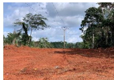
Clearing of line corridors in the East and West
