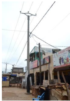
Yaoundé: Replacement of critical wooden poles with concrete poles in Emana and its surroundings
